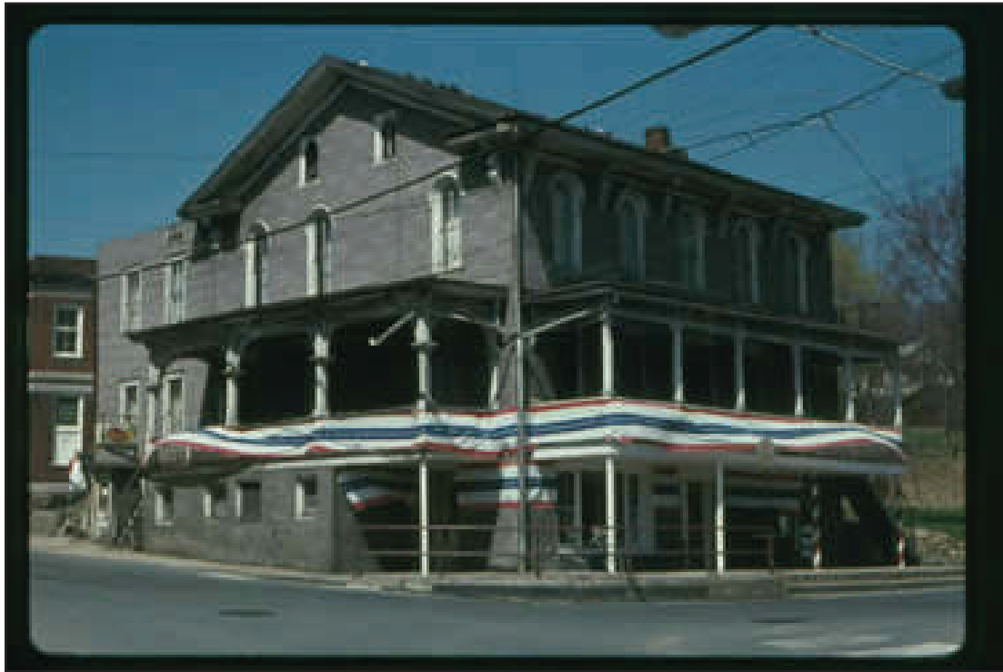
Figure 13: Montgomery Hotel. (Source:Montgomery Borough Website).
